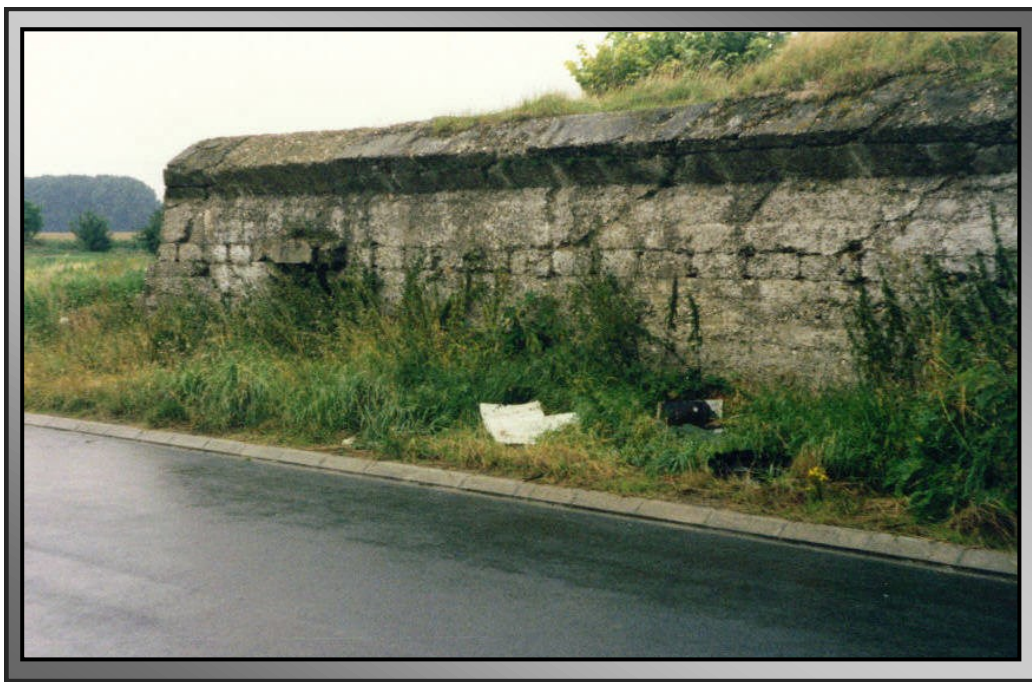
GERMAN CONCRETE BUNKER NEAR ROEUX
